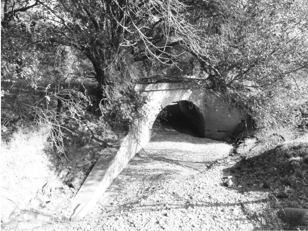
The old Railroad (?) bridge crossing Poppy Creek (built in 1909).
